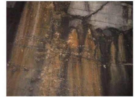
State assessment - extremely poor - HIGH RISK significant damages - ruined concrete - water flow
