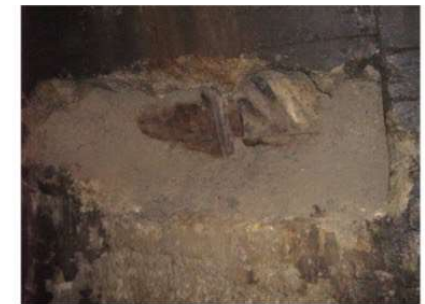
State assessment - extremely poor - HIGH RISK - caverns that punch the lining
