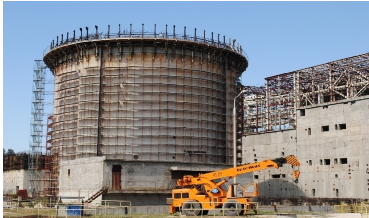
Image from during the assessment of the existing structures
